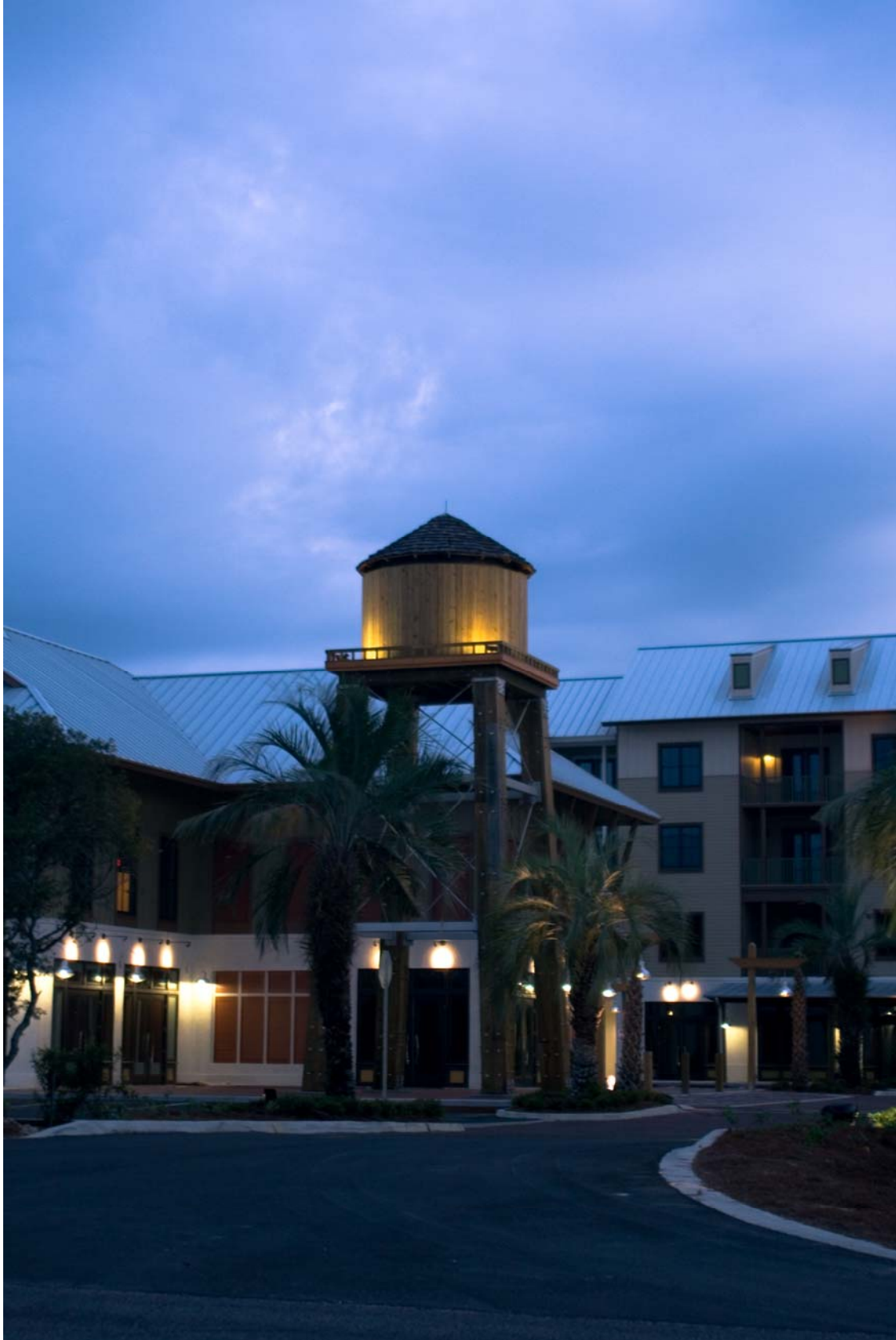
View of R1 & Water Tower
