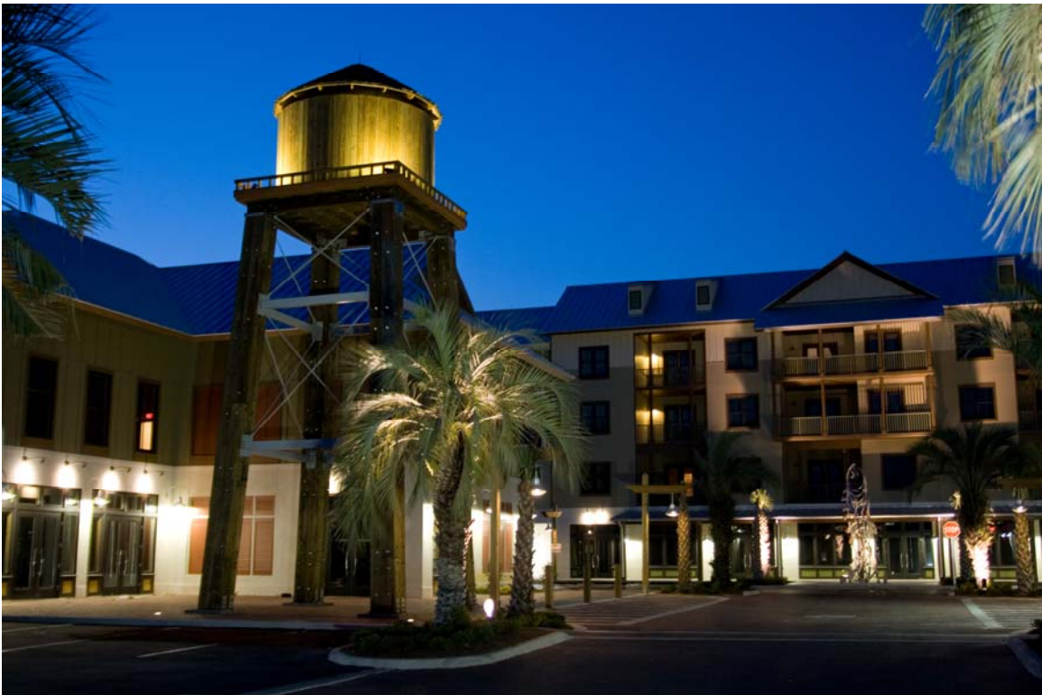
The Water Tower at night.
